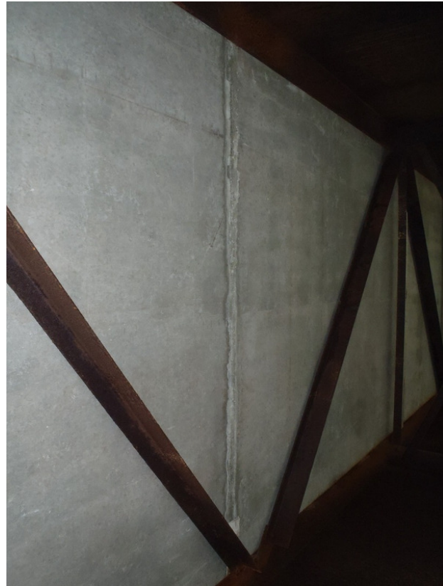
Figure 16: Typical underside of deck panels.
