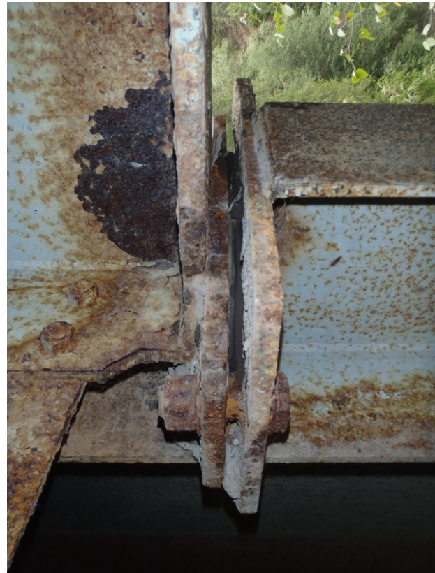
Figure 35: Pier 2 downstream bearing - Note condition of painted steel.
