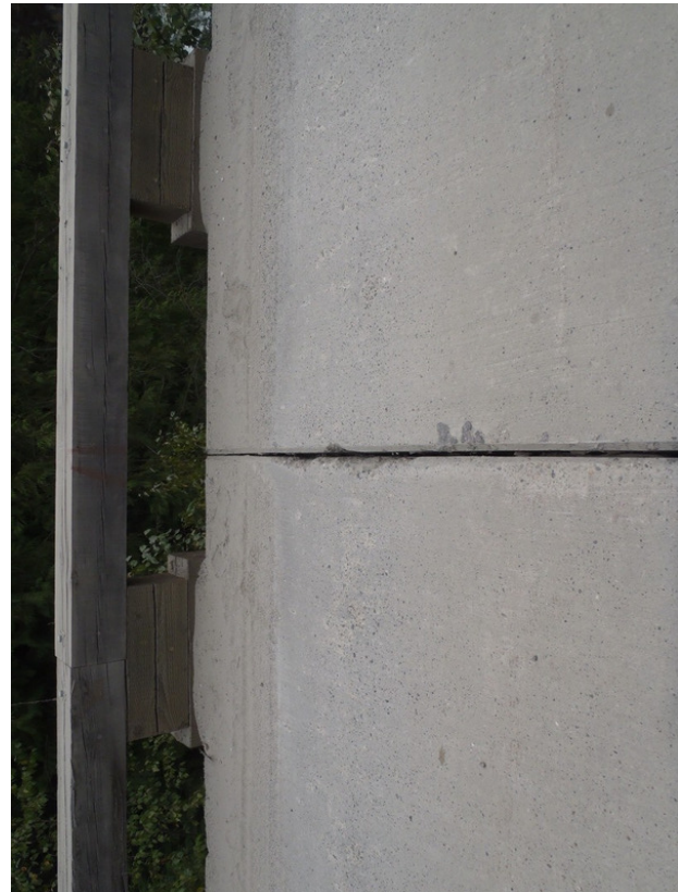
Figure 15: Typical condition of expansion joint.
