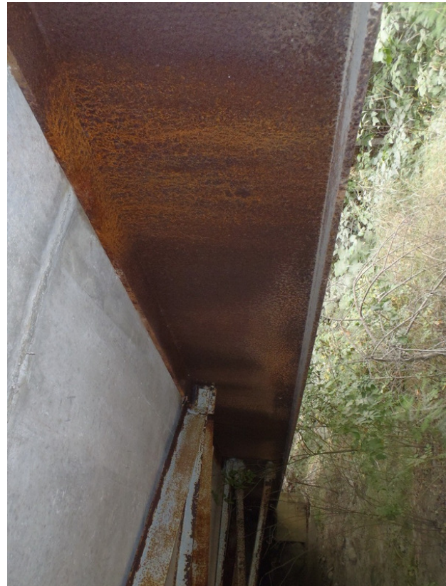
Figure 19: Typical interior face of girders - Span 3 girder 1 shown.
